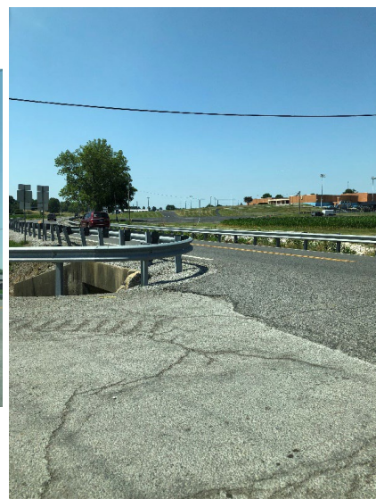
On KY 1176 looking south at US 60
